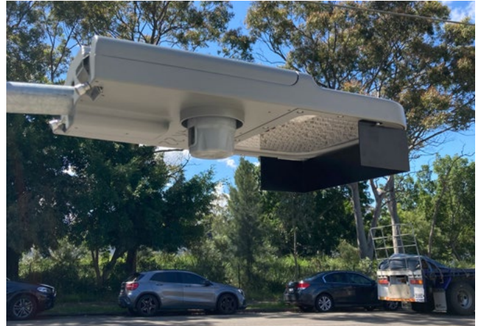
Front fitting attachment (VLEDVMF)
